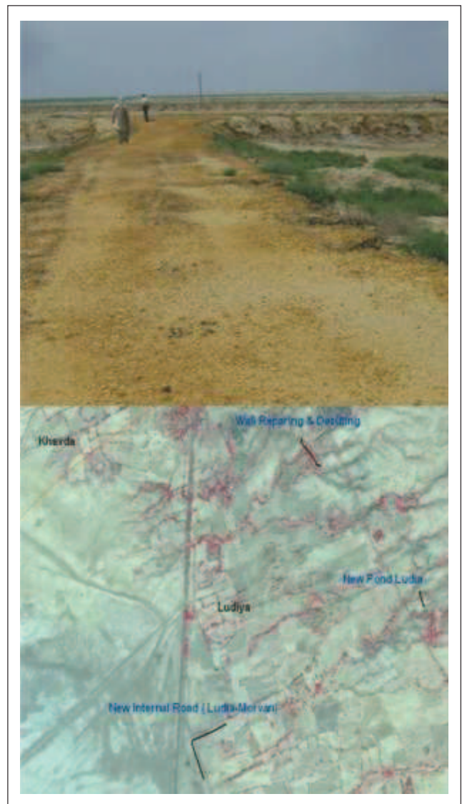
Figure 7: Mapping of Roads connectivity, wall repairing and desilting of pond
