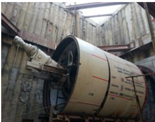
Figure 4: TBM at launching shaft
