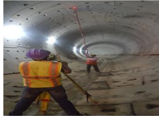
Figure 27: Final wriggle survey
