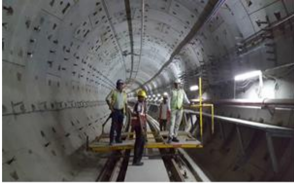
Figure 28: Schedule of Dimensions (SOD) checking in tunnel
