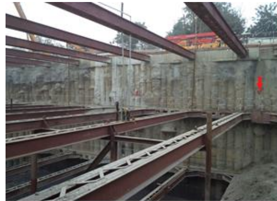
Figure 8: Targets at launching shaft
