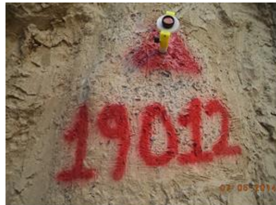
Figure 9: Glass prism target
