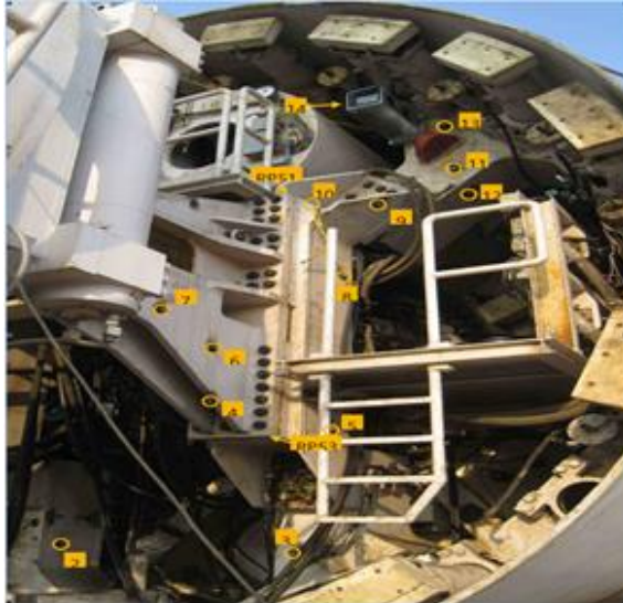
Figure 22: TBM manual survey points
