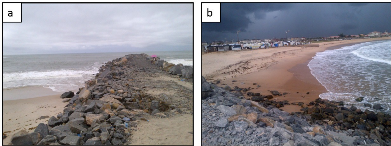
Figure 10: (a) A view down the length of one of the groins (b) Ongoing erosion alongside one of the groins constructed on the Lagos coast (Field survey, October 4, 2017)
